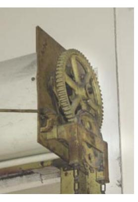
Before retrofitting, most fire doors have complex systems of mechanical gearing, governing devices and release mechanisms.
