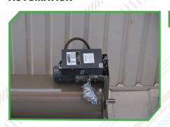
A variety of motor operators are available to optimize the efficiency of our rolling door and grille products. A full line of controls and accessories can ensure both safety and convenience.
